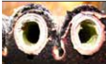
Scale buildup from untreated water.
